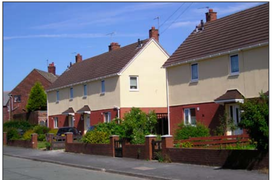
Below: After refurbishment
