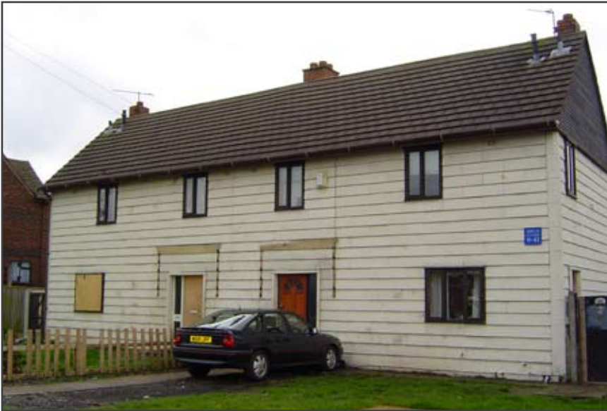
Left: Before refurbishment
